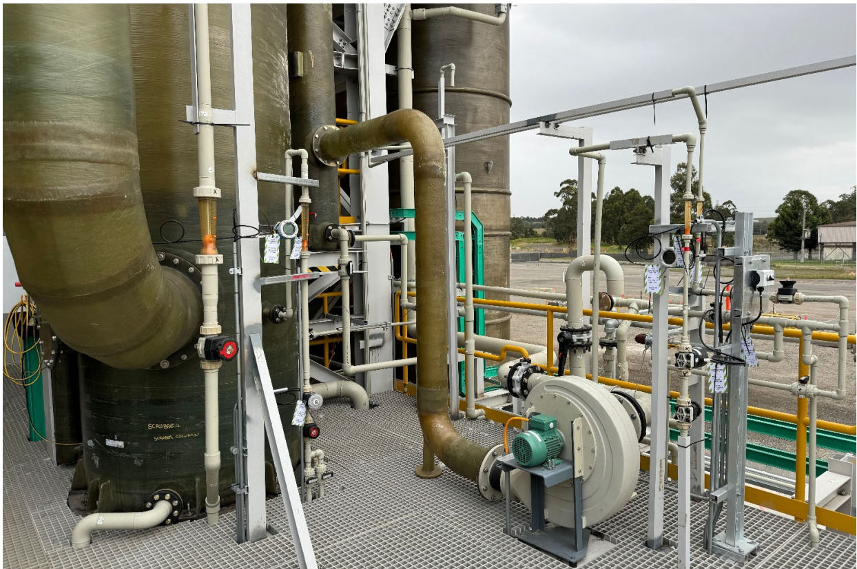
Figure: Spray Roaster construction complete
