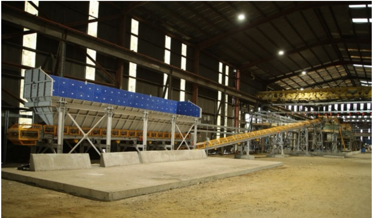
Figure: Magnesite Hopper, Bag Breaker, and Fly Ash areas ready for operations
