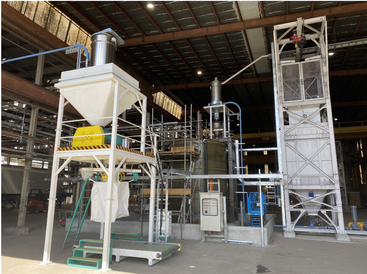
Figure: Magnesium Bagging Plant
