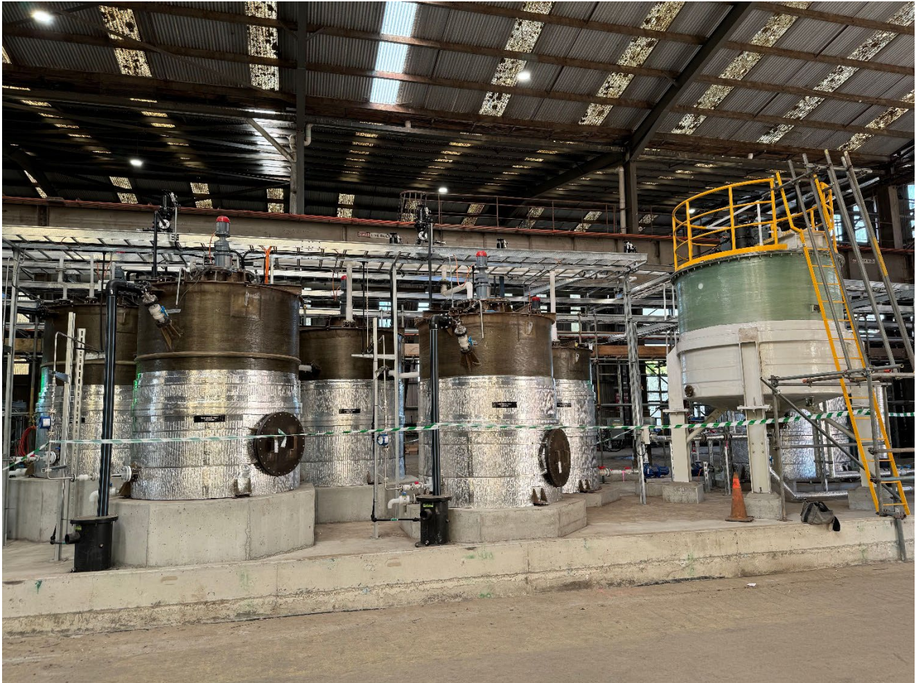
Figure: Hydromet area construction complete and commissioned
