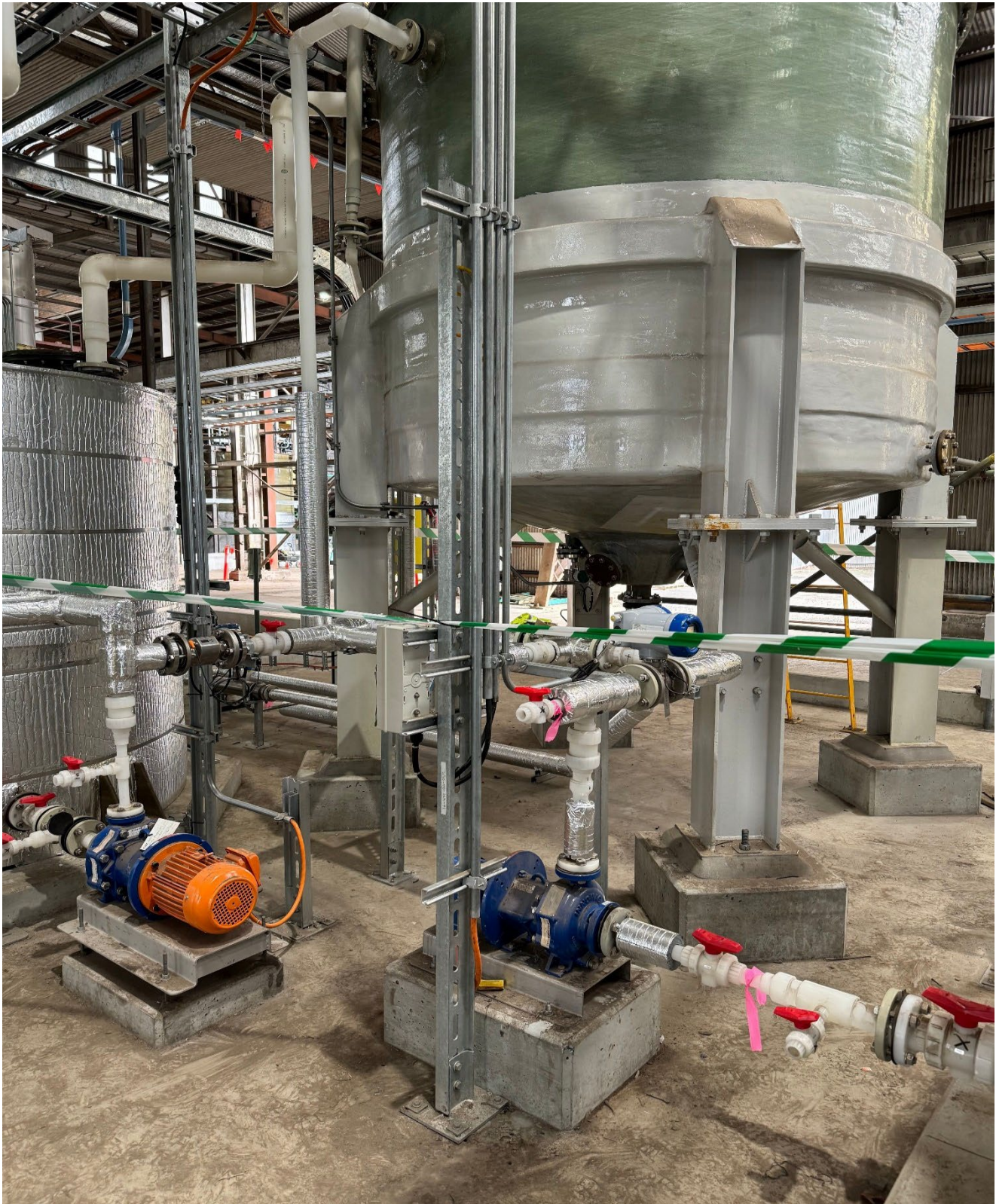
Figure: Hydromet piping, and insulation completed and commissioned.
