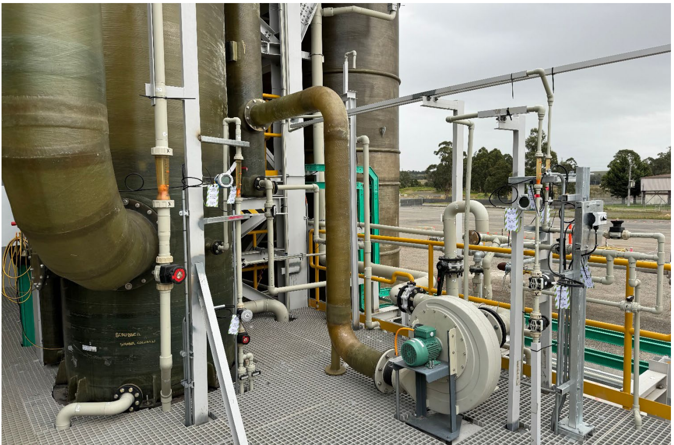
Figure: Spray Roaster construction complete
