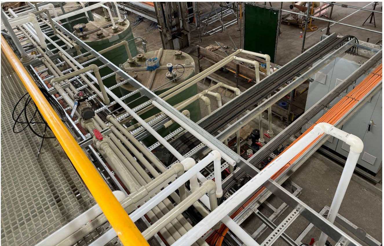
Figure: Filtration area complete with all piping, hydraulics and electrics installed
