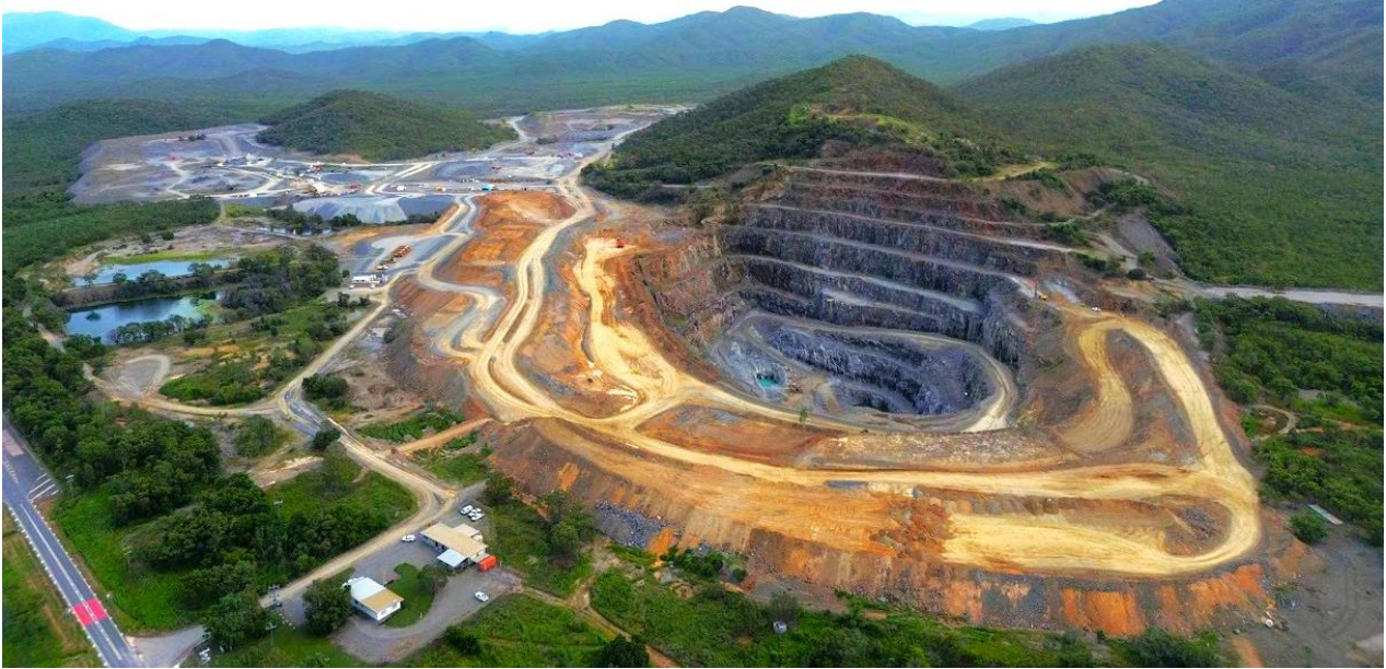
Picture above: The Andy White Open Pit end of March 2024 with the noise and visual bund in the foreground
