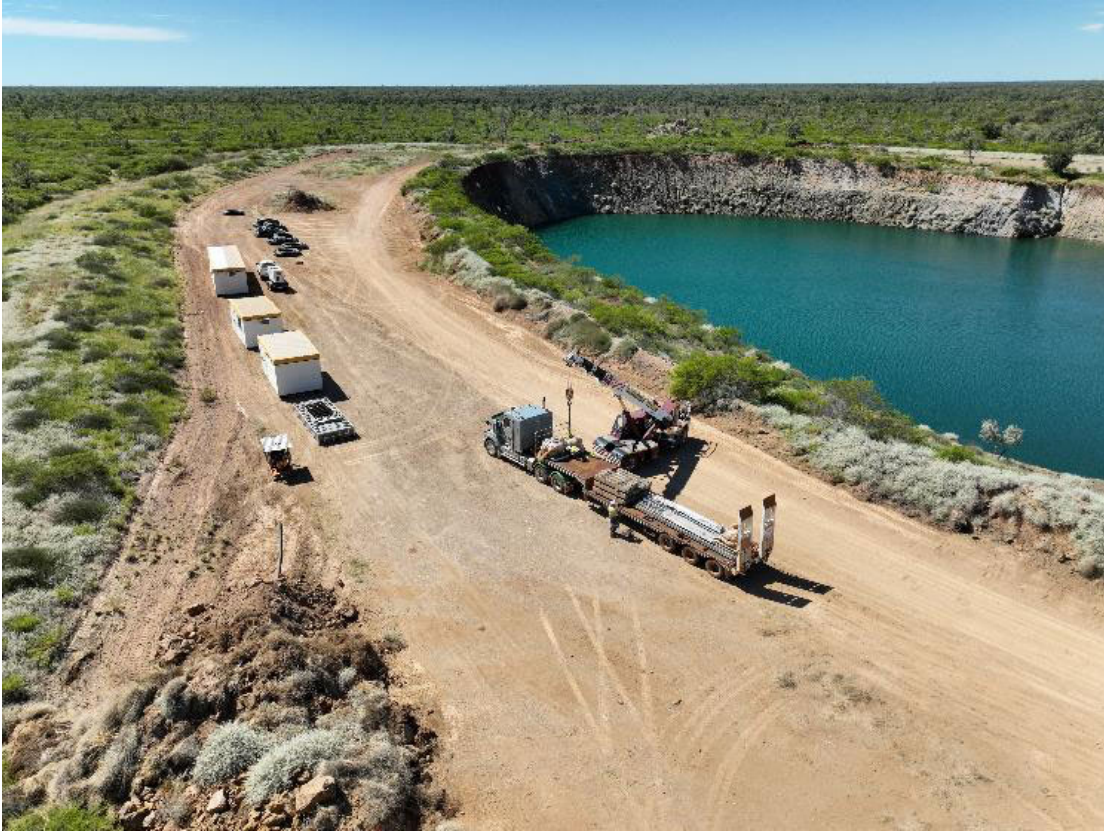
Figure 5. Wallace North office, workshop and fuel facility preparation adjacent to water source at Wallace South Pit. Image taken 23 April 2024.
