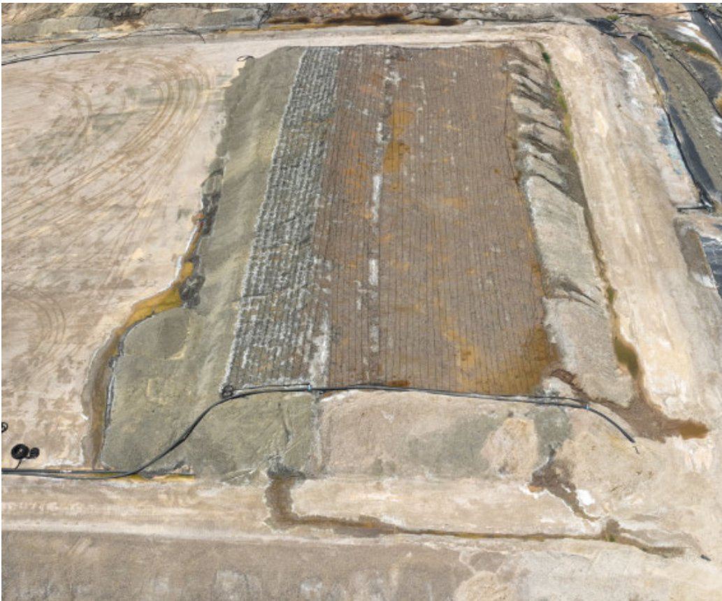
Figure 6. Great Australia Heap Leach Pad 5 advancing with new stacked material from existing stockpiled ore on left of heap.
