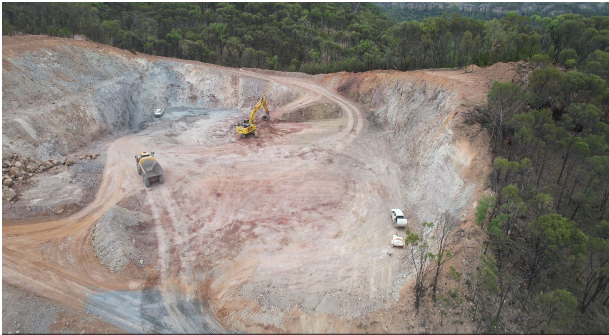
Sherwood West Pit 4 progress
