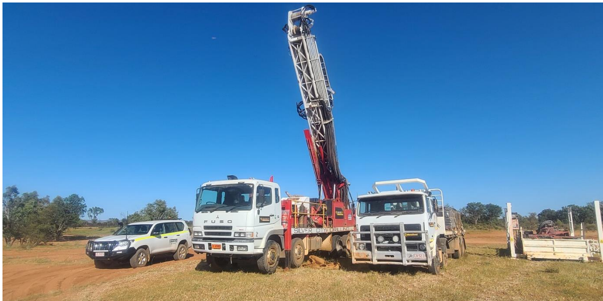
Figure 1 – Drill rig on site at salt bush bore near Silver King.
