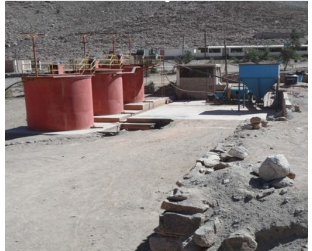
Current 40 tpd plant – approval to upgrade to 200tpd
