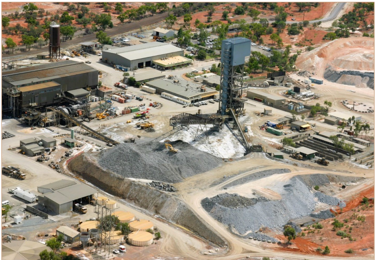
Endeavor Mine, Cobar NSW, Australia
