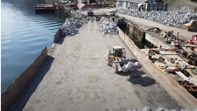
Figure 4-314: Typical rock barge being loaded by front-end loader
