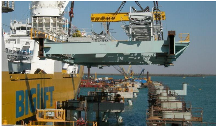
Figure 6: Modulated wharf construction using HLS
