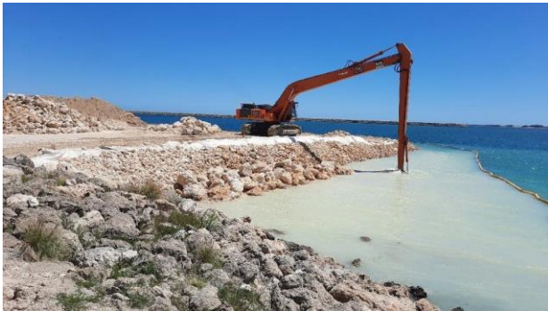
Figure 18: Installation of primary and secondary rock armour on top of geofabric
