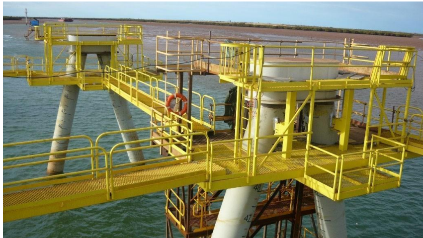
Figure 29: Pile bracing and walkways installed
