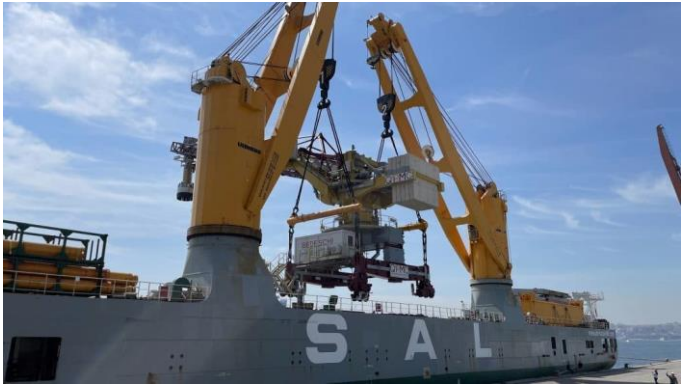
Figure 3637 : HLS lifting a fully assembled shiploader
