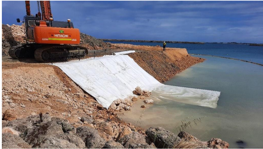
Figure 17: Installation of geofabric on top of fill
