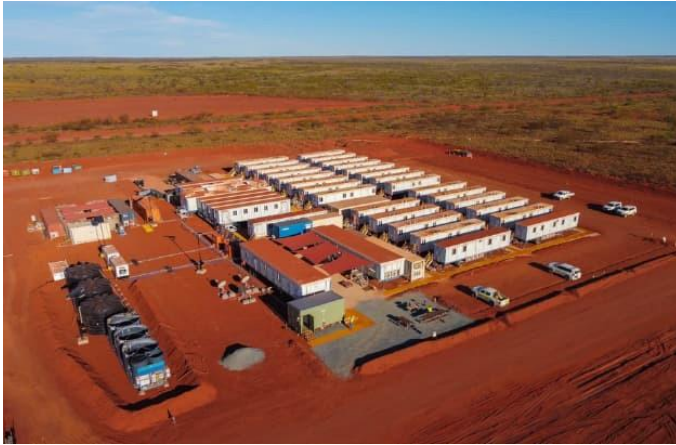
Figure 2425: Typical construction camp using transportable buildings
