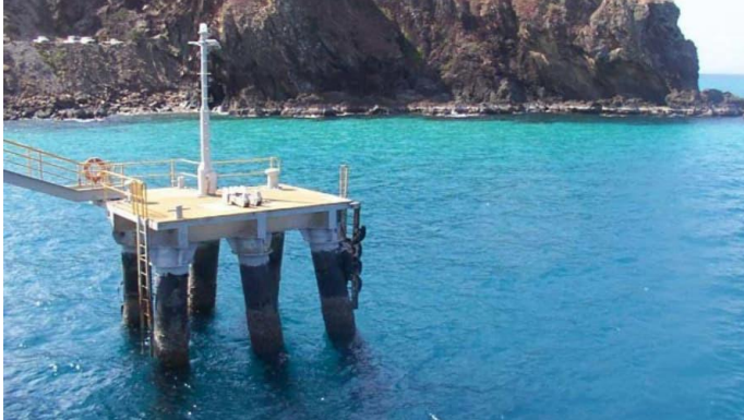
Figure 2930: Mooring dolphin structure consisting of 6 raked piles
