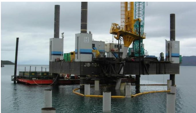
Figure 2627: Pile top drill rig and piling frame mounted to SEMP
