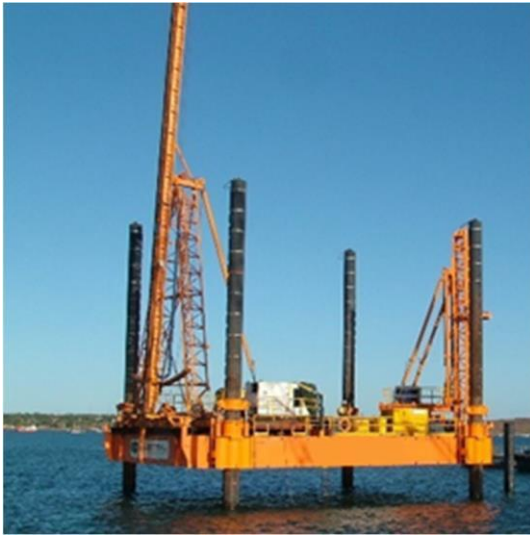
Figure 21: SEMP used to install mooring piles.
