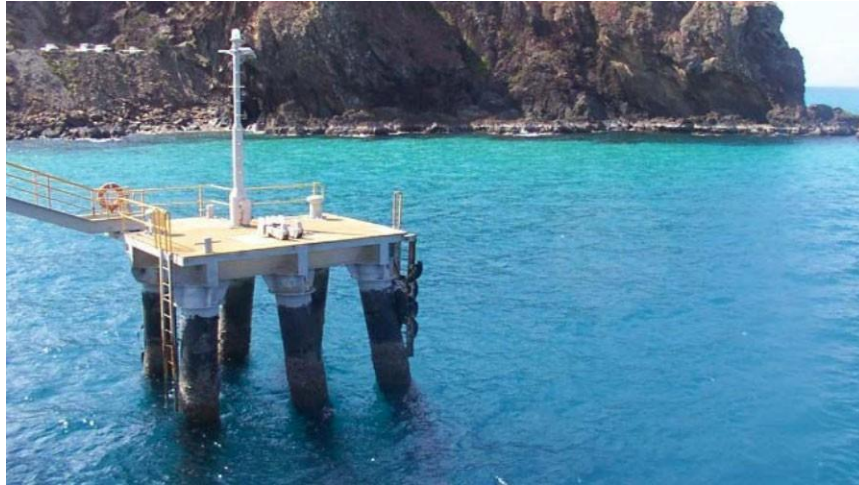
Figure 30: Mooring dolphin structure consisting of 6 raked piles
