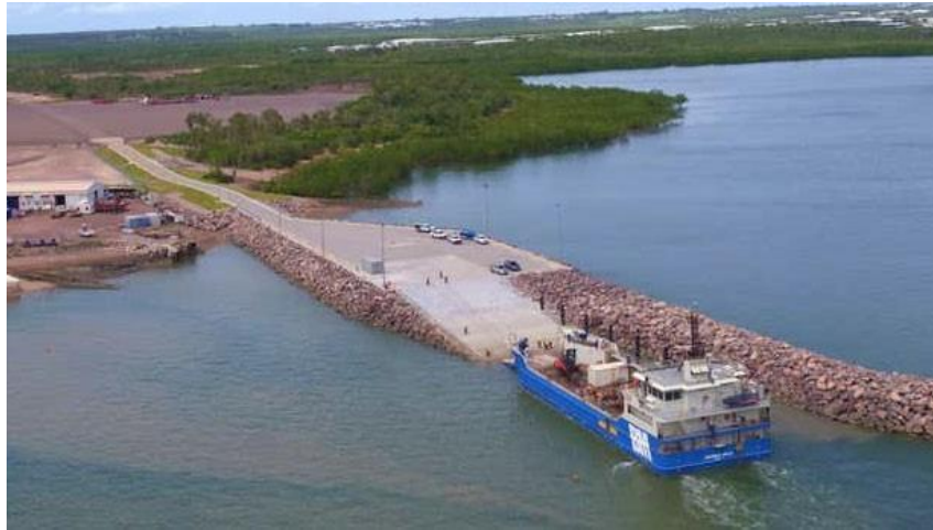
Figure 23: Landing ramp for RORO vessel or landing craft
