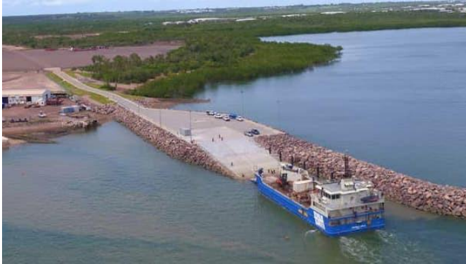
Figure 2223: Landing ramp for RORO vessel or landing craft
