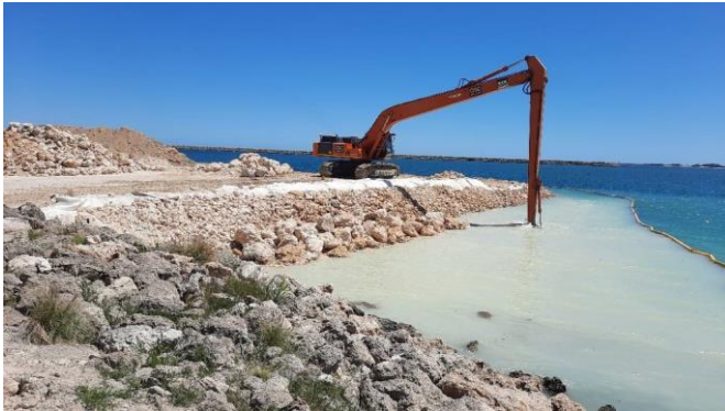
Figure 17: Installation of geofabric on top of fill
