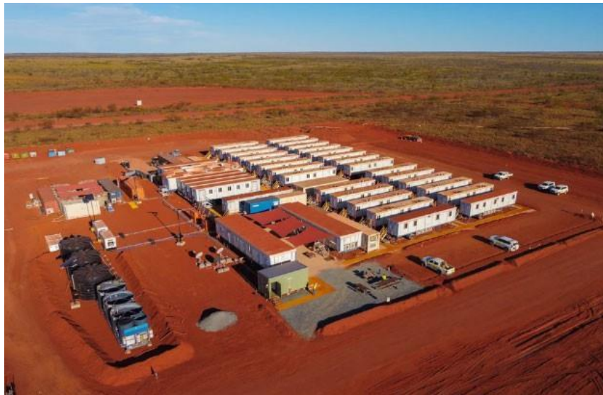
Figure 25: Typical construction camp using transportable buildings
