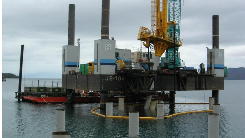
Figure 27: Pile top drill rig and piling frame mounted to SEMP
