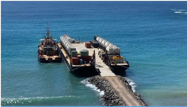
Figure 5: Temporary barge offloading facility
