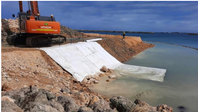
Figure 4516: FEL, excavator and dump truck working to place fill for typical armoured rock wharf
