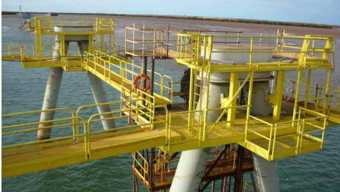
Figure 2829: Pile bracing and walkways installed
