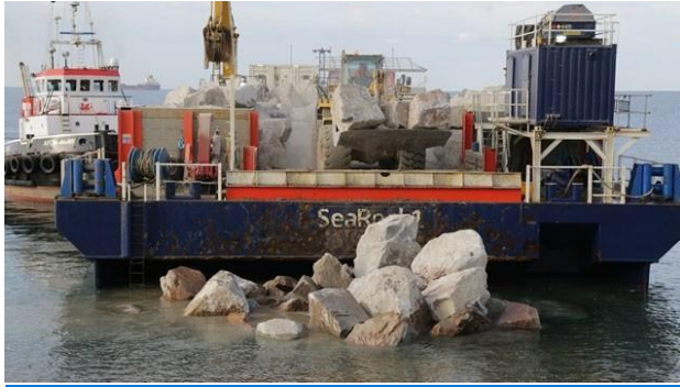
Figure 4-415: Typical rock barge being offloaded by front-end loader
