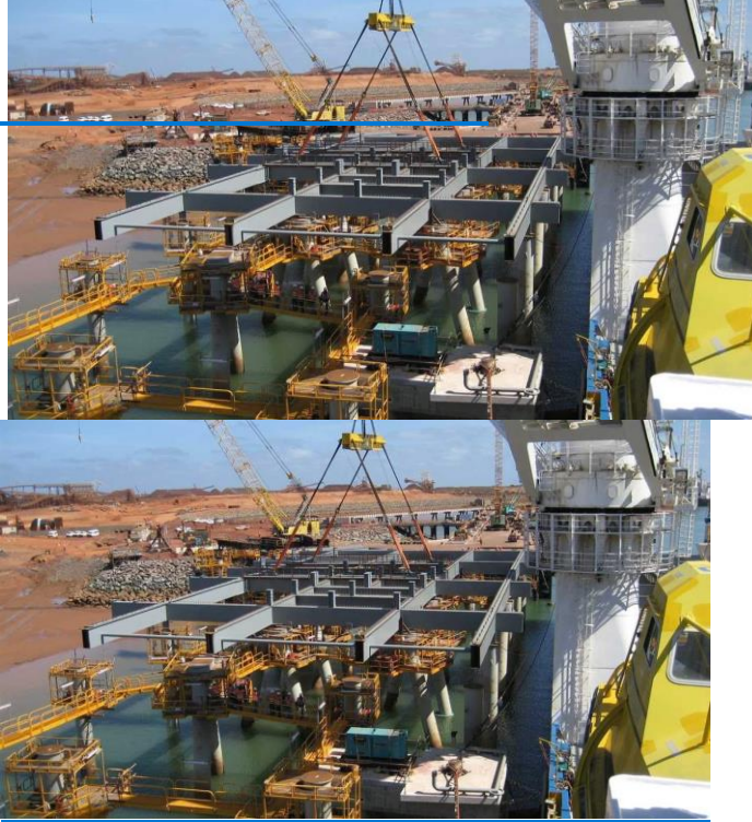
Figure 3432: HLS installing prefabricated deck modules
