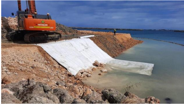
Figure 16: Installation of geofabric on top of fill
