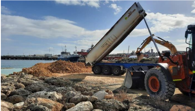
Figure 4516: FEL, excavator and dump truck working to place fill for typical armoured rock wharf
