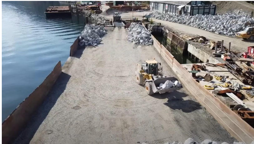
Figure 14: Typical rock barge being loaded by front-end loader
