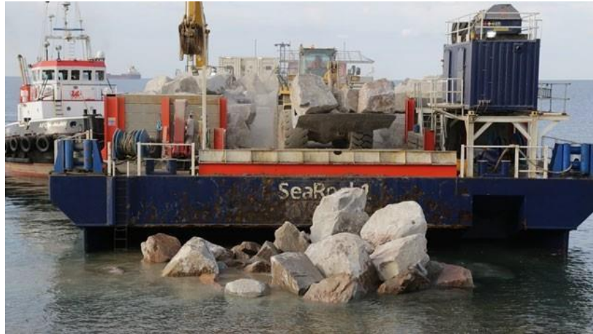
Figure 15: Typical rock barge being offloaded by front-end loader
