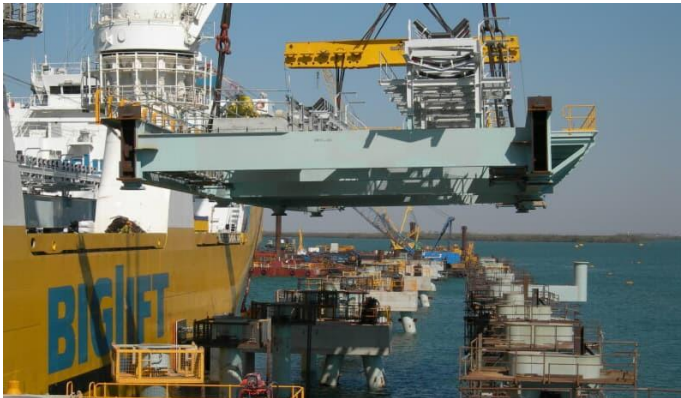
Figure 6: Modular wharf construction using HLS
