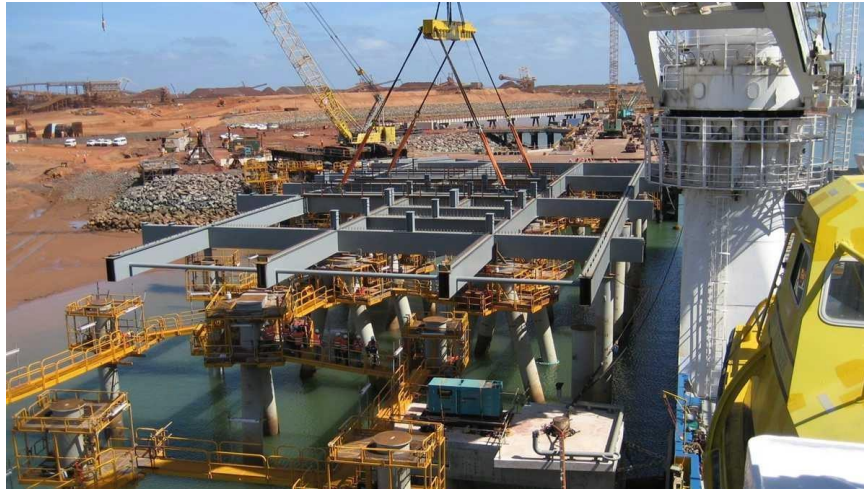
Figure 32: HLS installing prefabricated deck modules
