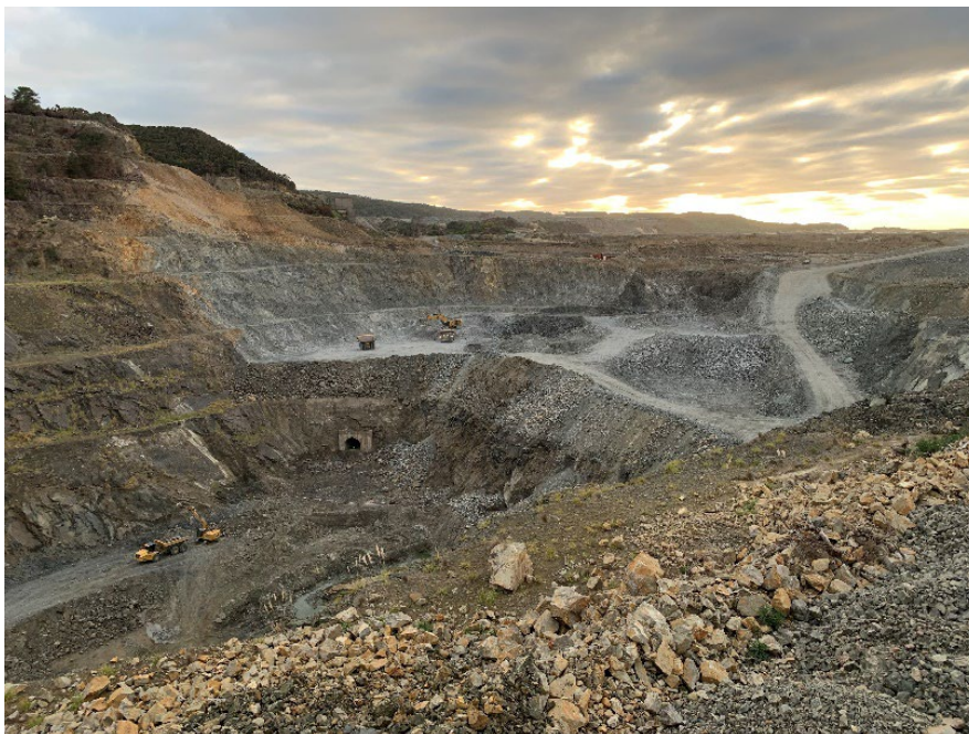
Figure 1 - Dolphin Open Cut Stage 1 Bench Development at RL-30m, above high-grade C-lens - May 2024
