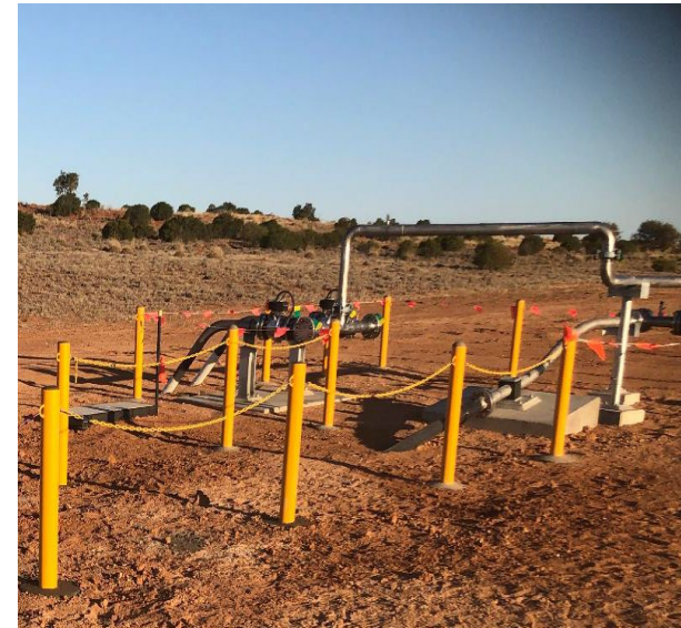
Odin -1 pipeline tie-in point to Vali-Beckler pipelines
