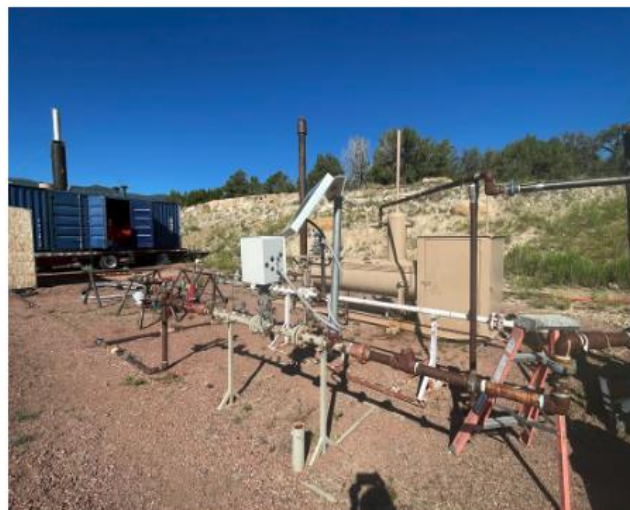
Images 1 & 2: The Pathfinder 1 well (L) and the gas connection point linking to the generator (R)
