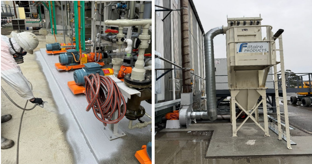
Figure: Acid resistant epoxy coating for Spray Roaster (left) and SCM Dust Collector & Stack installed (right)
