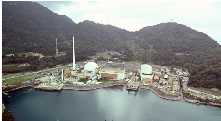
Angra is Brazil's only nuclear plant. (Image courtesy of International Atomic Energy Agency Brazil / Flickr Commons .)
