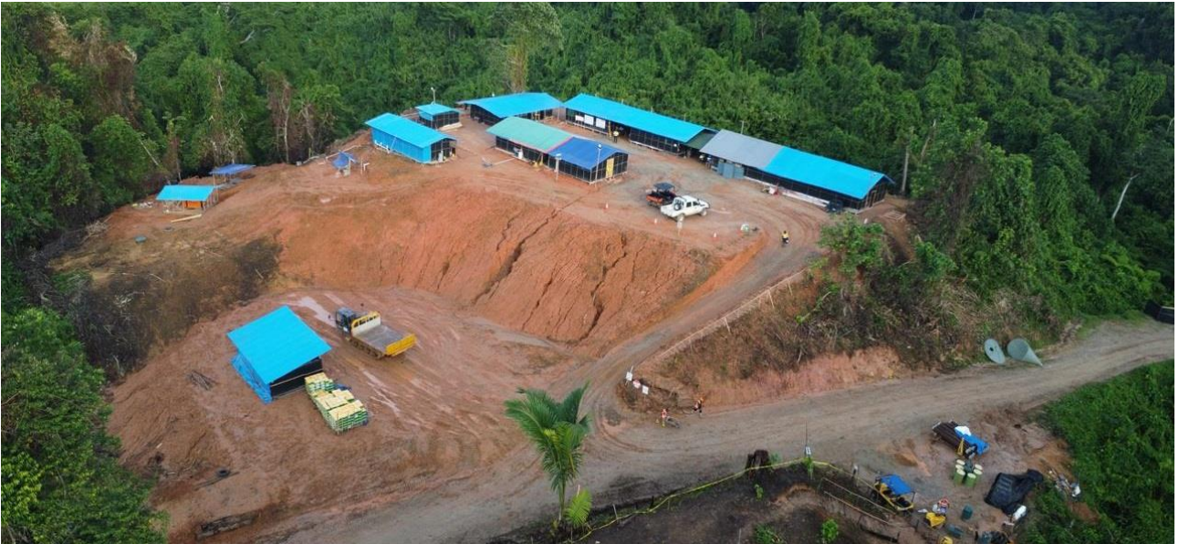
Figure 5 Chachu'lu field camp & laydown area, June 2024.
