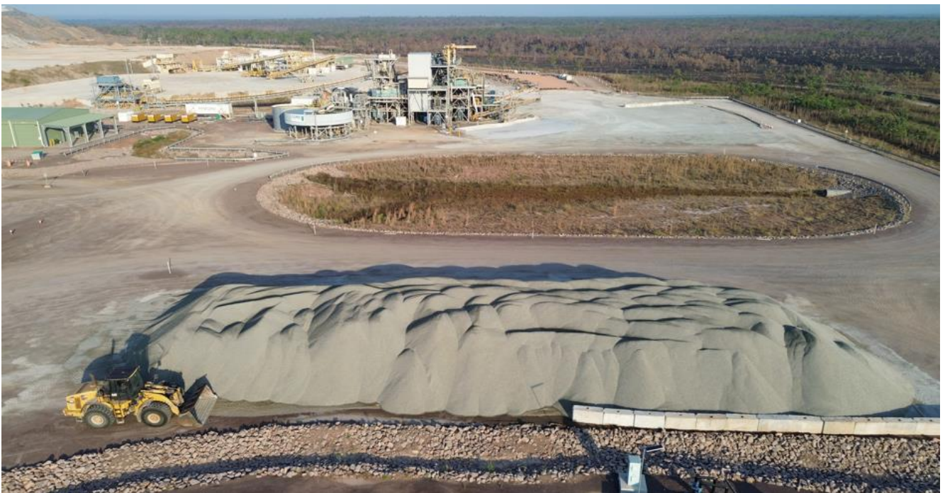
Figure 2 Spodumene Concentrate Stockpile
