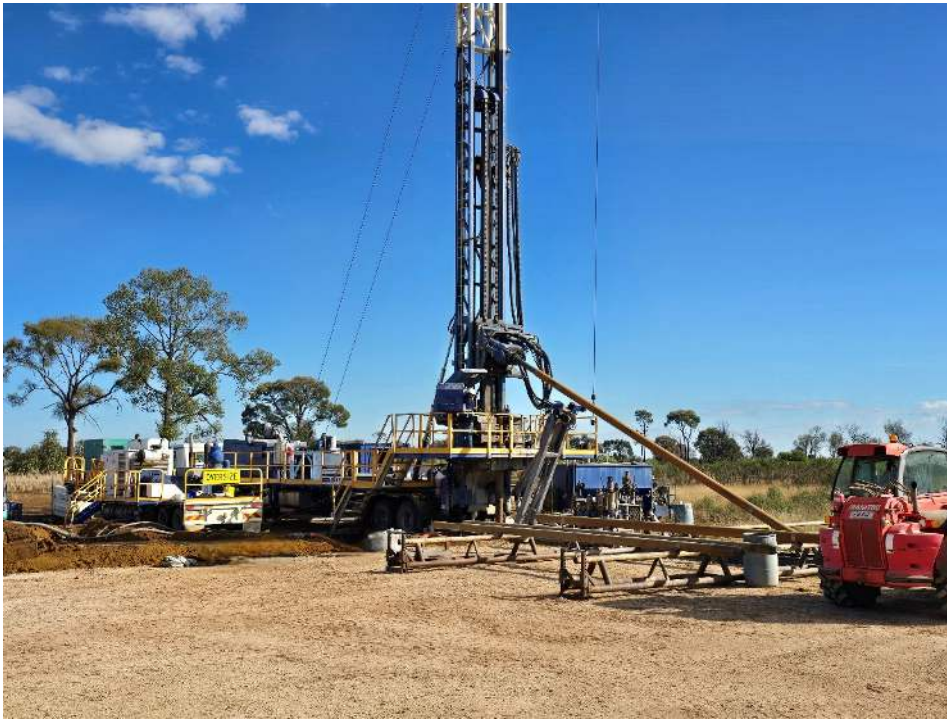
Figure 1-Drilling of the Canyon-1 Water Bore
