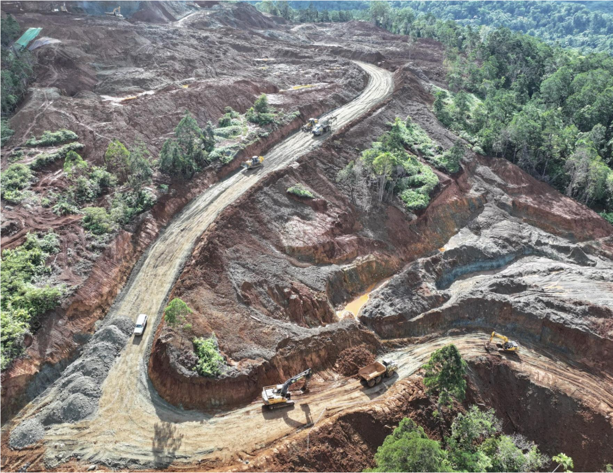
Kolosori haul road being repaired – now completed
