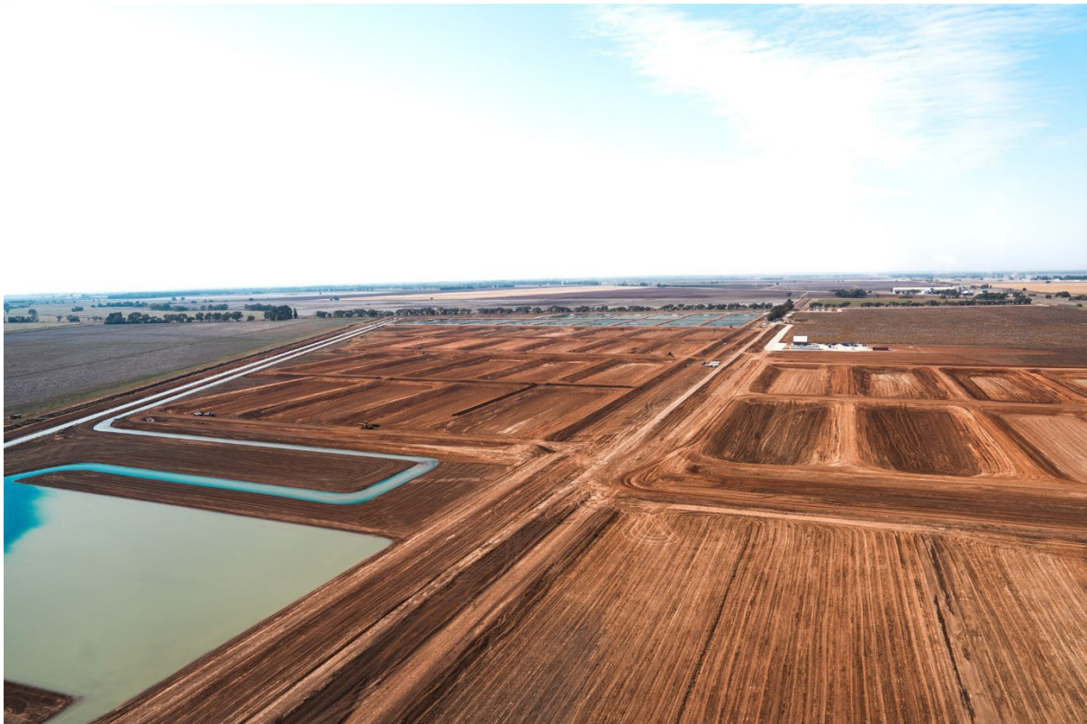
Construction at Stanbridge Site May 2024
