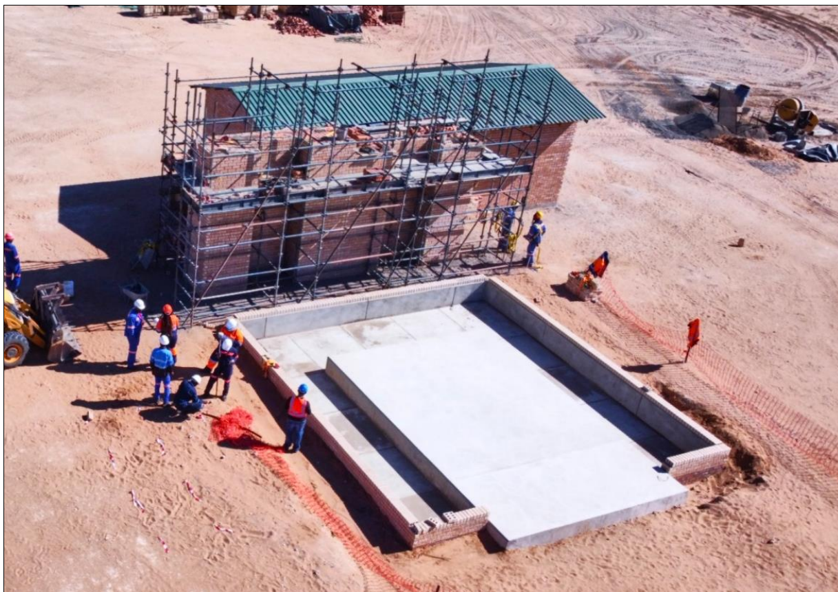
Control room and transformer plinth construction at the Lesedi substation – July 2024
