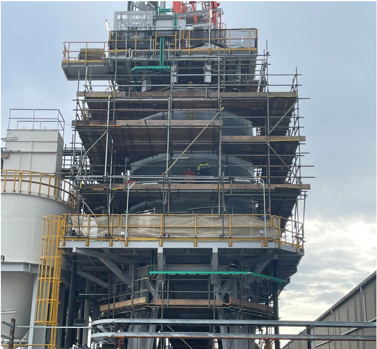
Figure: Spray Roaster scaffold completed ready for insulation works
