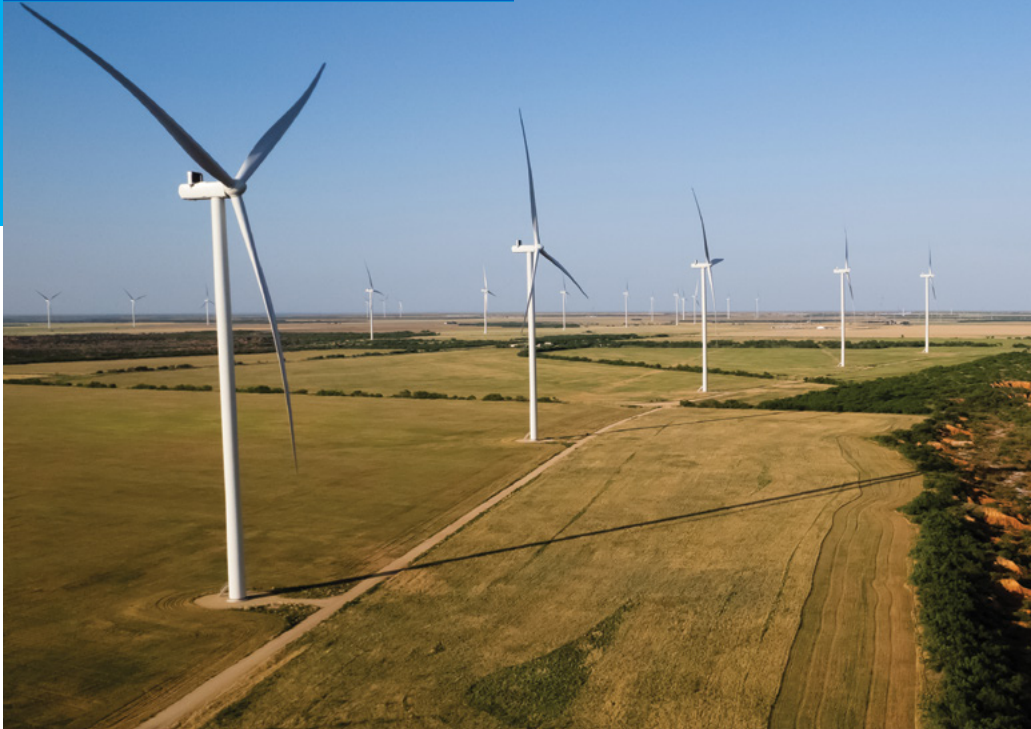
Longroad Energy 243MW El Campo wind farm, Texas
