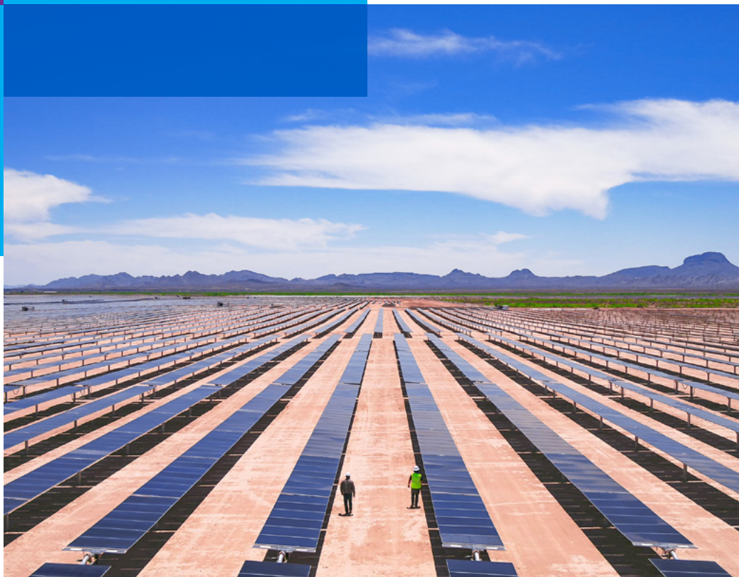
Longroad Energy's Sun Streams 2, solar farm, Arizona
