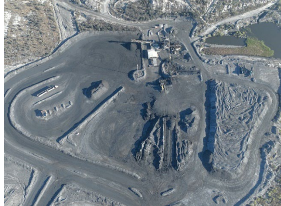
Blair Athol Coal Handling and Preparation Plant
