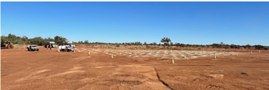
Figure 1 & 2: The 1st Blast shot being loaded in readiness for firing at Wallace North
