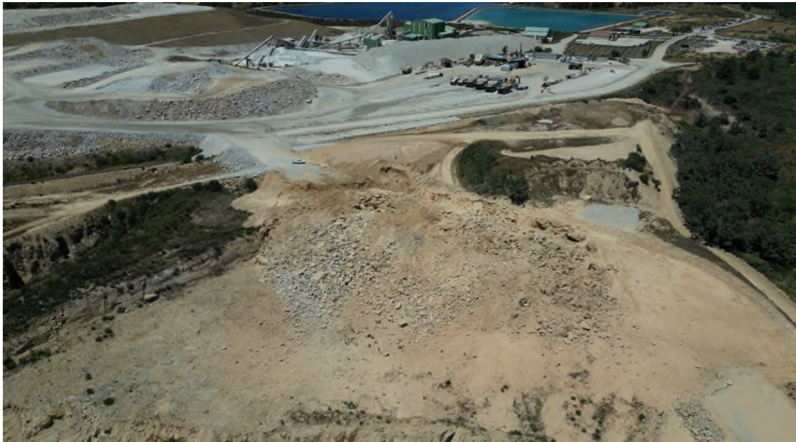
Surface blast during the Phase 6 Works
