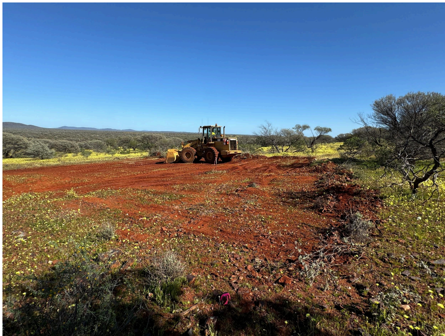
Figure 01: Earthworks commencing at the Remorse Target
