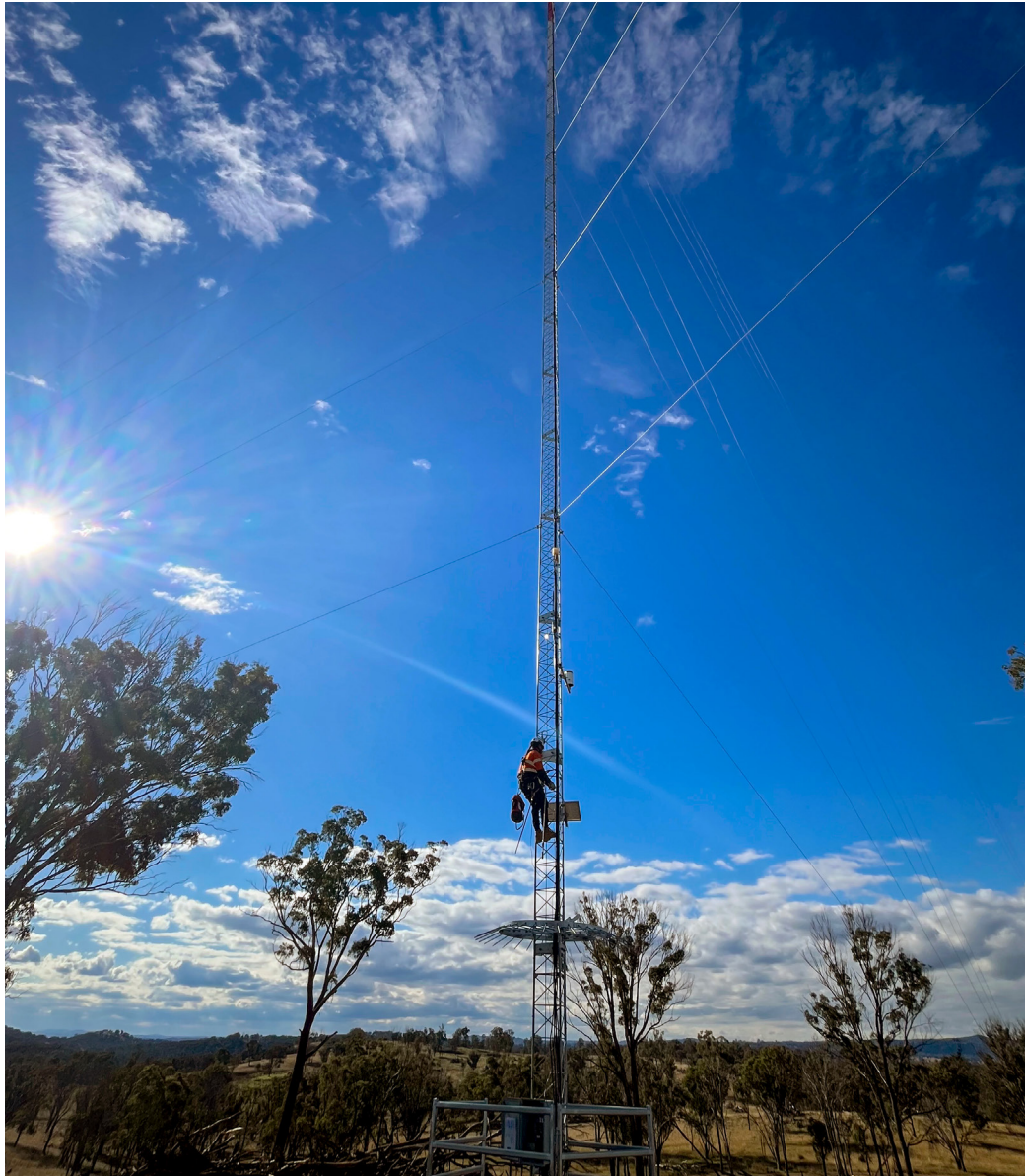
▲ A meteorological mast at Northern Tablelands Wind Farm at Warrane, gathering data to help identify the best locations for turbines.
