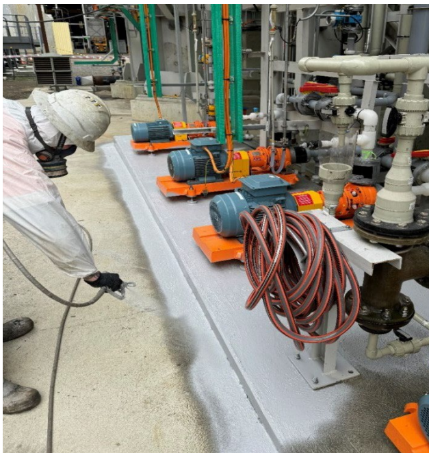
Acid resistant epoxy coating for Spray Roaster (left) and SCM Dust Collector & Stack installed (right)
