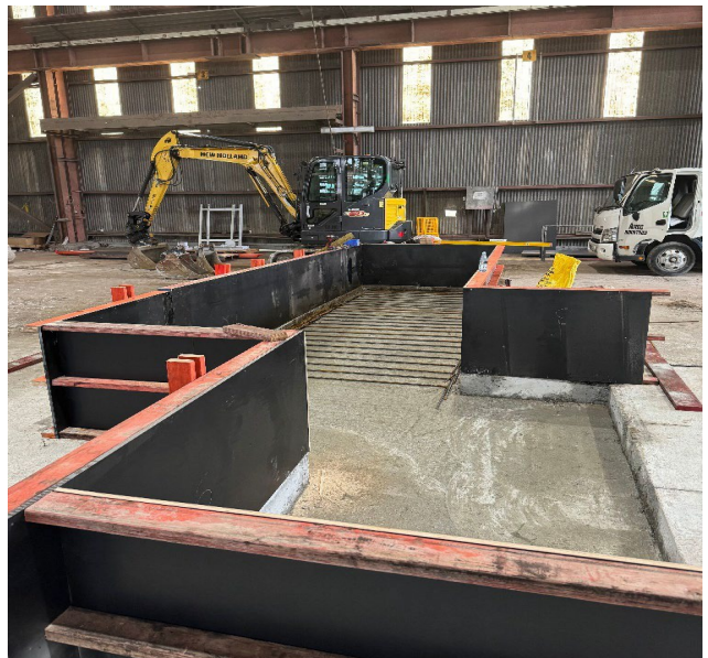
Ferrosilicon Bag Breaker erection (left) and Briquetting Ball Mill civil works (right)
