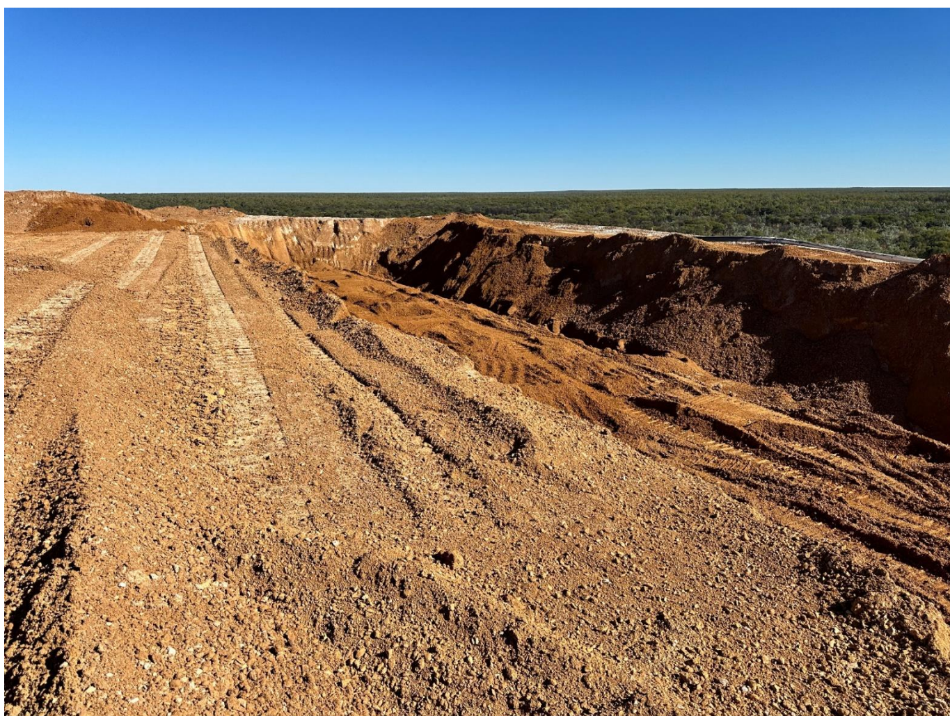
Figure 1. Pad 2/3 Re-Mine Operation at commencement.
