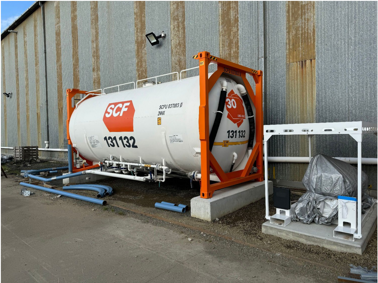
Figure: Quicklime piping installation in progress
