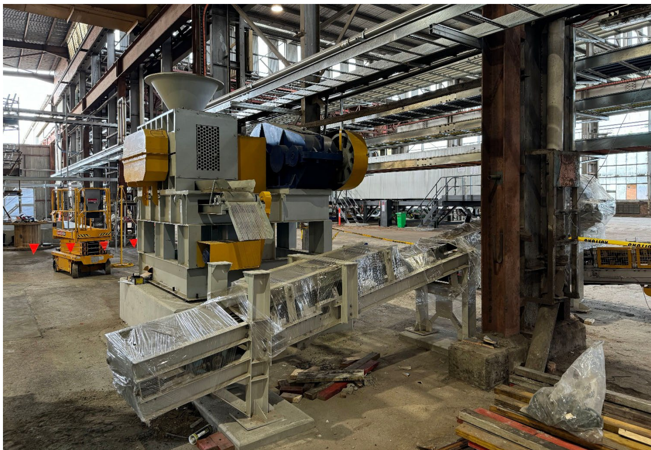
Figure: Briquette civil formwork in progress (top) Briquetting machine, conveyor placed on completed concrete foundations (bottom)
