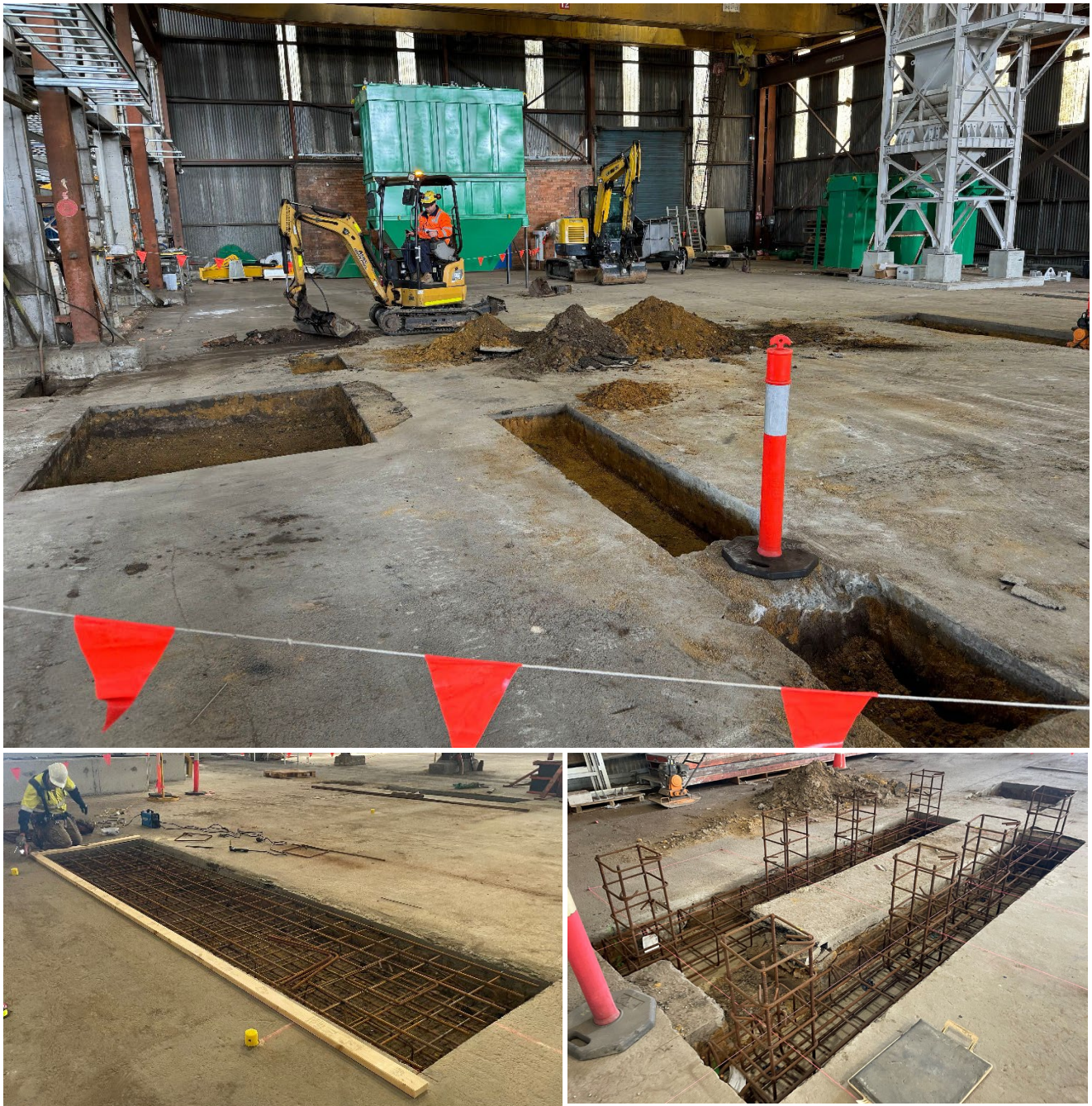
Figure: Briquette civil work excavation and rebar works in progress
