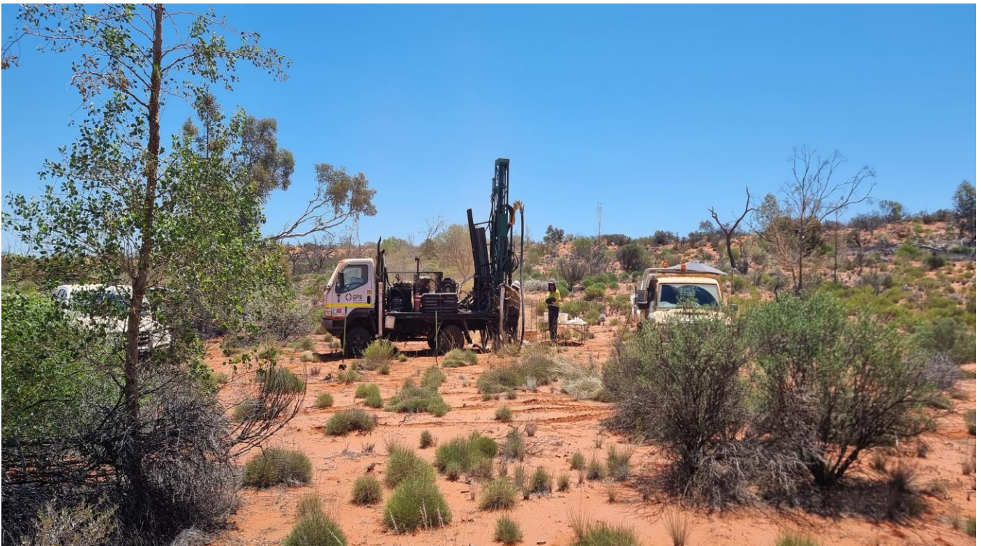
Fig 2 : Cyclone drilling program on site
