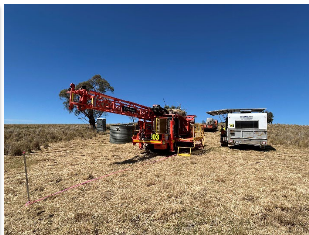
Figure 4: Drill Rig in position for first hole
