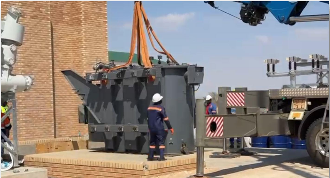
5MVA Transformer being hoisted into place at the Lesedi Substation – November 2024
