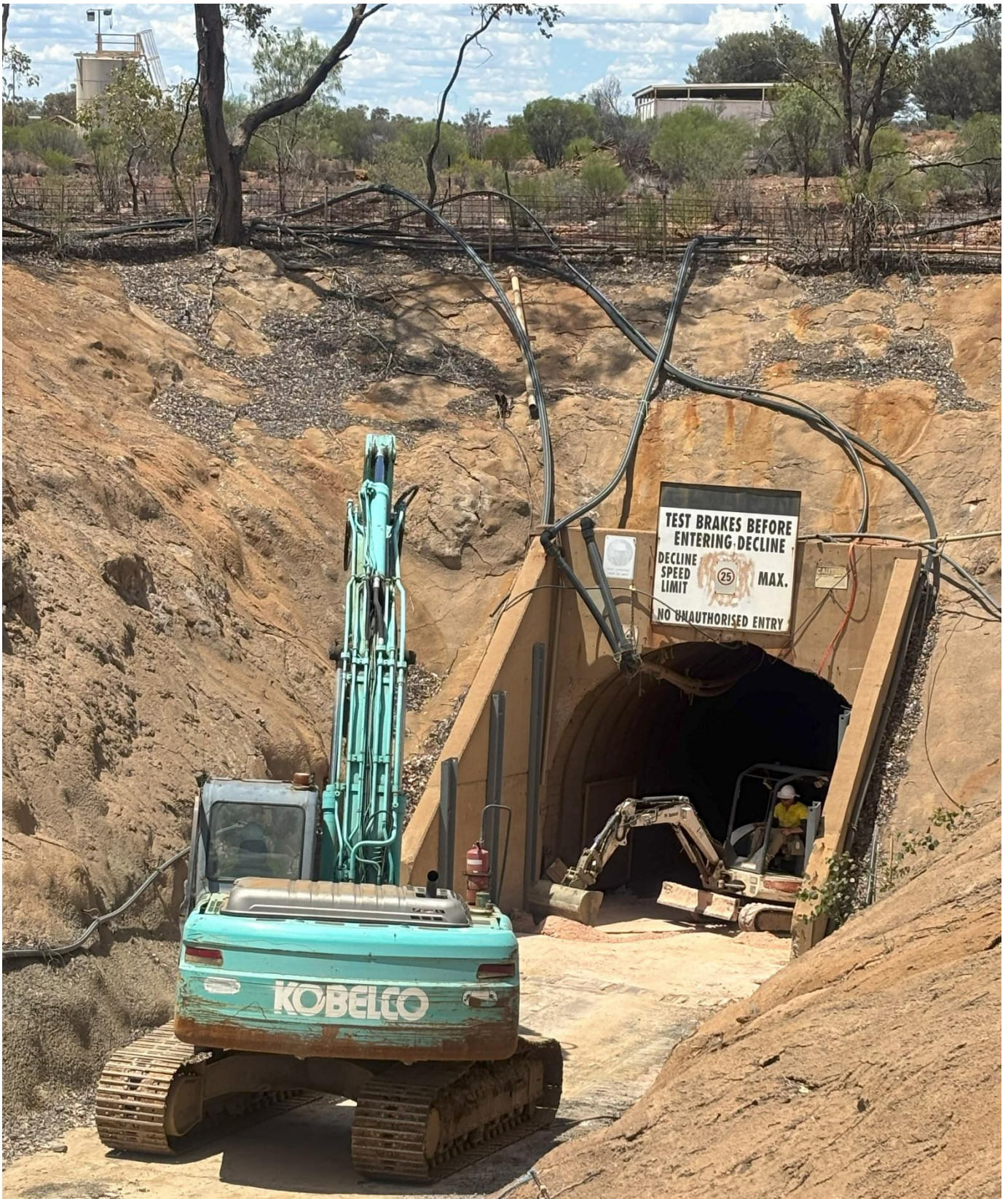
Figure 3: Modification of the mine portal entrance to allow access for larger 65t trucks
