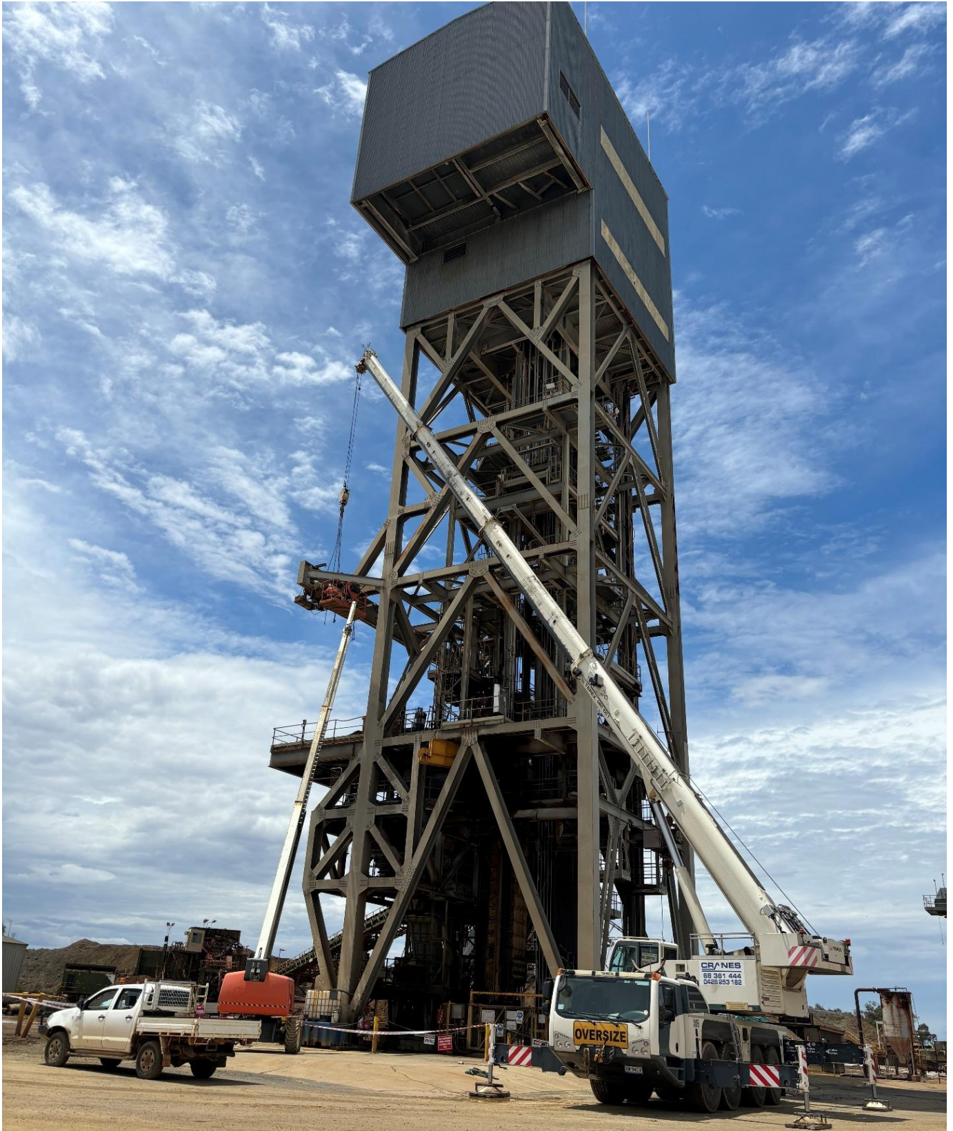
Figure 2: Refurbishment and re-certification of headframe gantry crane.
