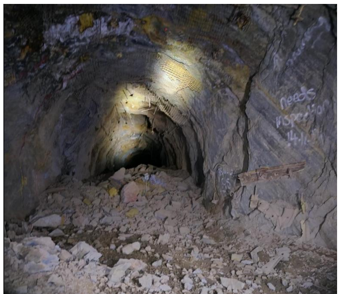
Figure 4. Level 1: Charged (LHS) & blasted (RHS) to establish ventilation to Upper North Lode (UNL).
