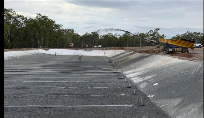
Lining of bio-retention ponds
