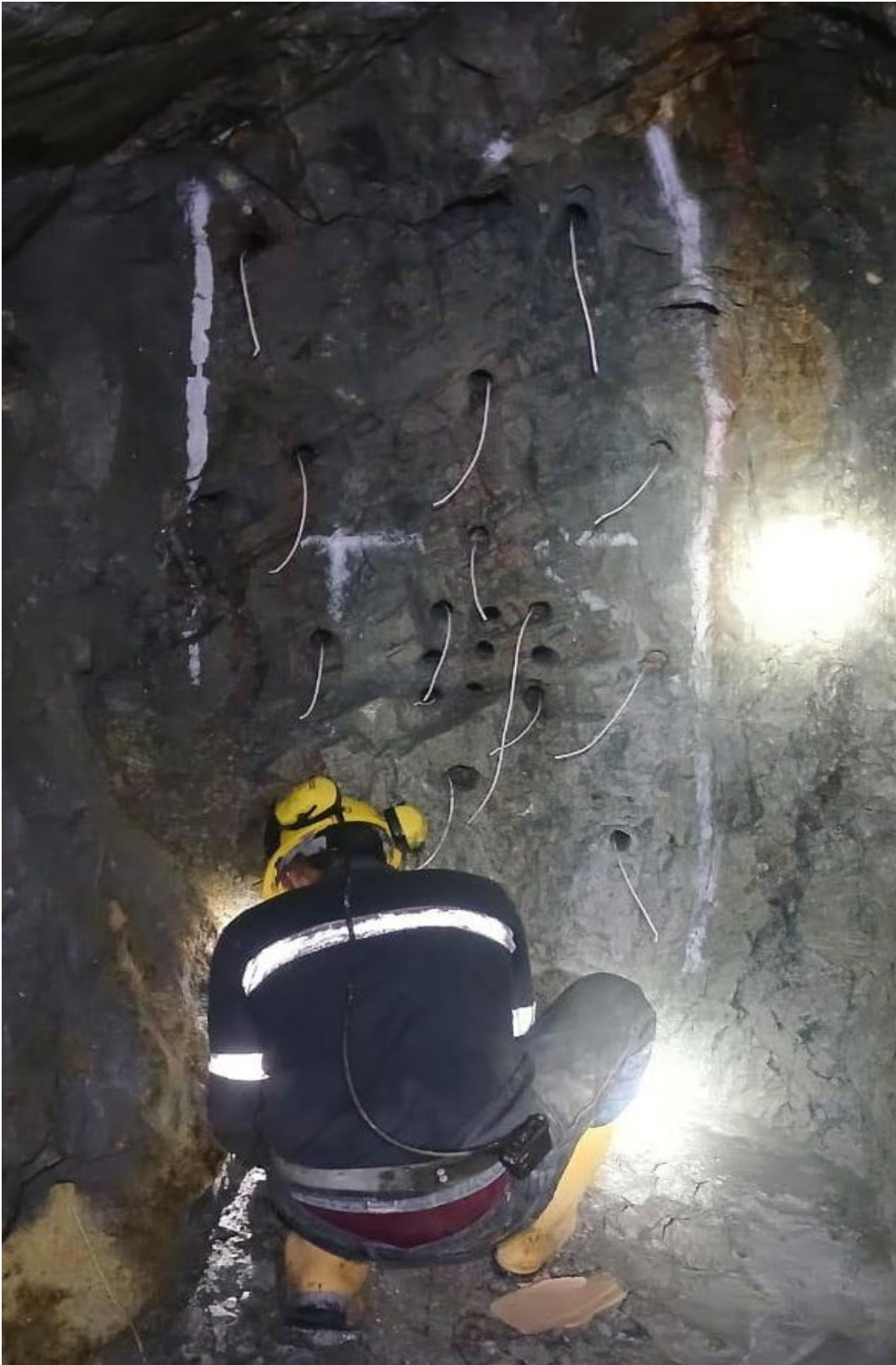
Image 2: Charges being set in underground development at the Santa Barbara vein
