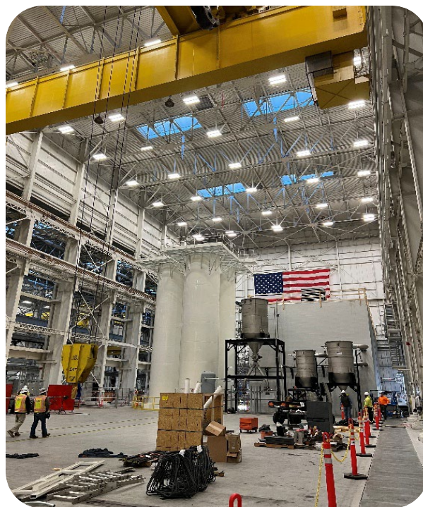
Figure 2 Silos - Raw Material Processing
