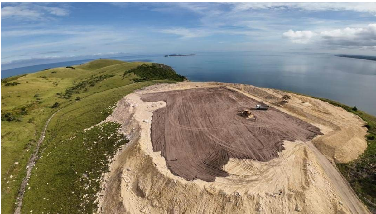
Image 3: Topsoiling being completed for the community sports field
