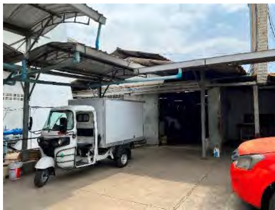
View of the single-storey laundry building
