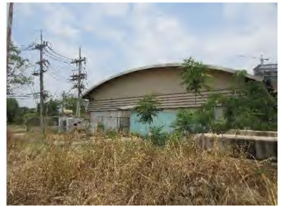
View of the single-storey power plant building
