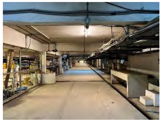
Internal view of the double-storey casino (Basement)
