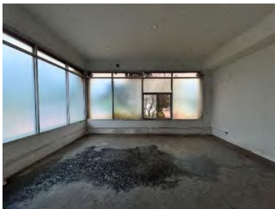
Internal view of the single-storey gymnasium
