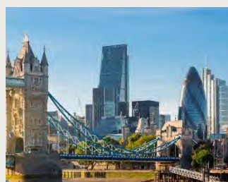
Valuation Leadenhall Building, London
