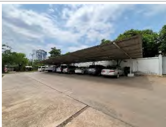
View of the open-sided car park
