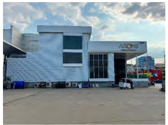
View of the double-storey restaurant
