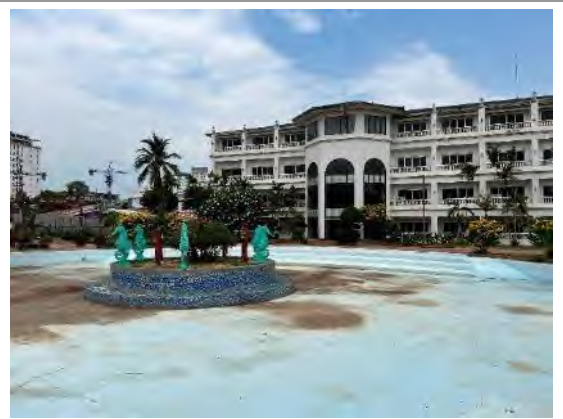
View of the swimming pool
