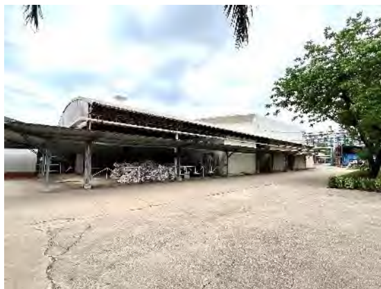
View of the single-storey warehouse 2
