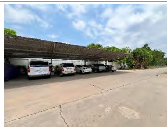
View of the open-sided car park
