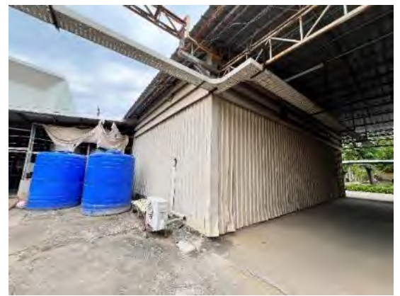
View of the single-storey warehouse 2
