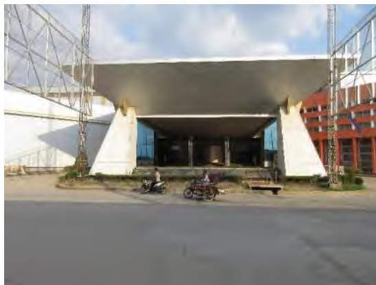
View of the single-storey casino (Casino 3)
