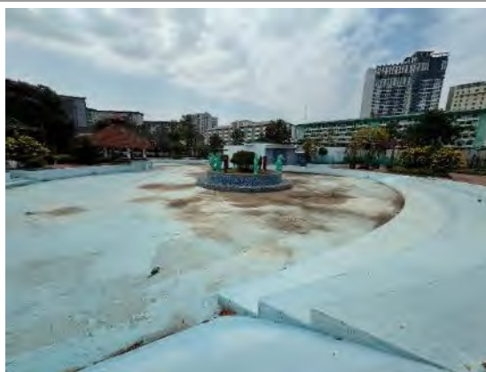
View of the swimming pool
