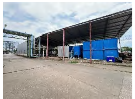
View of the single-storey water chiller building
