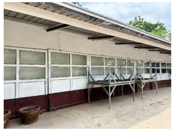
View of the single-storey warehouse 1
