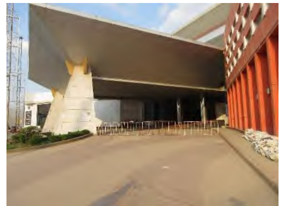
View of the single-storey casino (Casino 3)
