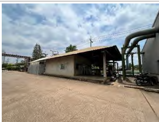
View of the single-storey water chiller control building
