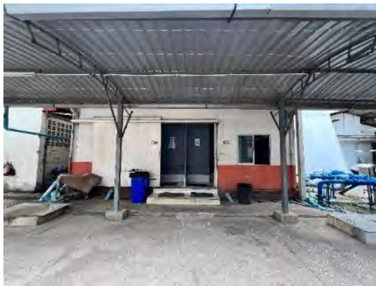
View of the single-storey male/female water closets (WCs)
