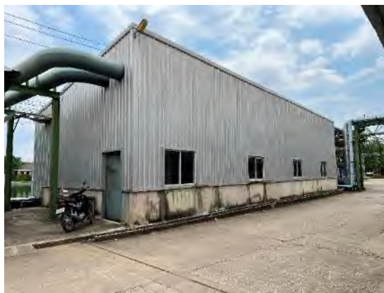
View of the single-storey water chiller building
