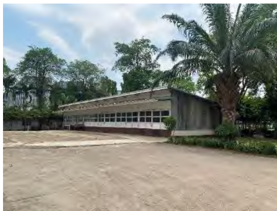
View of the single-storey warehouse 1
