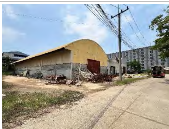
View of the single-storey warehouse 3
