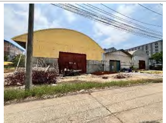
View of the single-storey warehouse 3
