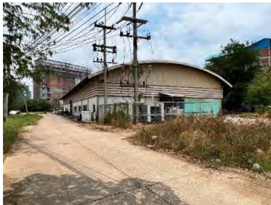
View of the single-storey power plant building
