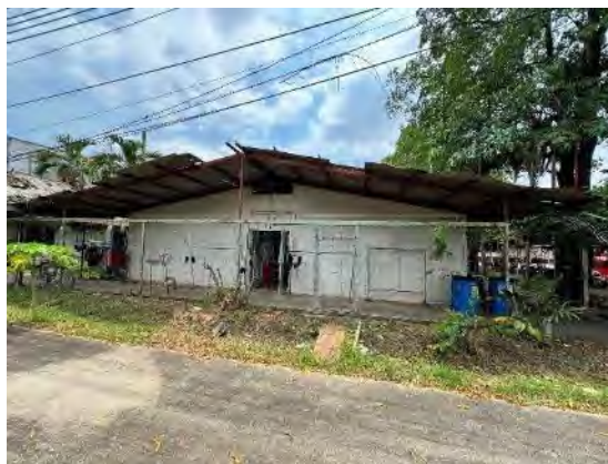
View of the two single-storey residence
