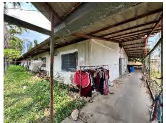
View of the two single-storey residence
