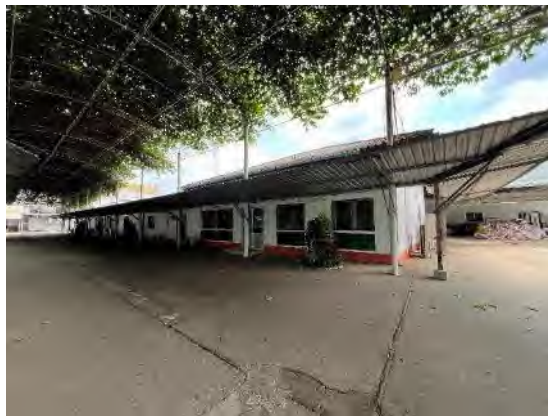
View of the single-storey office
