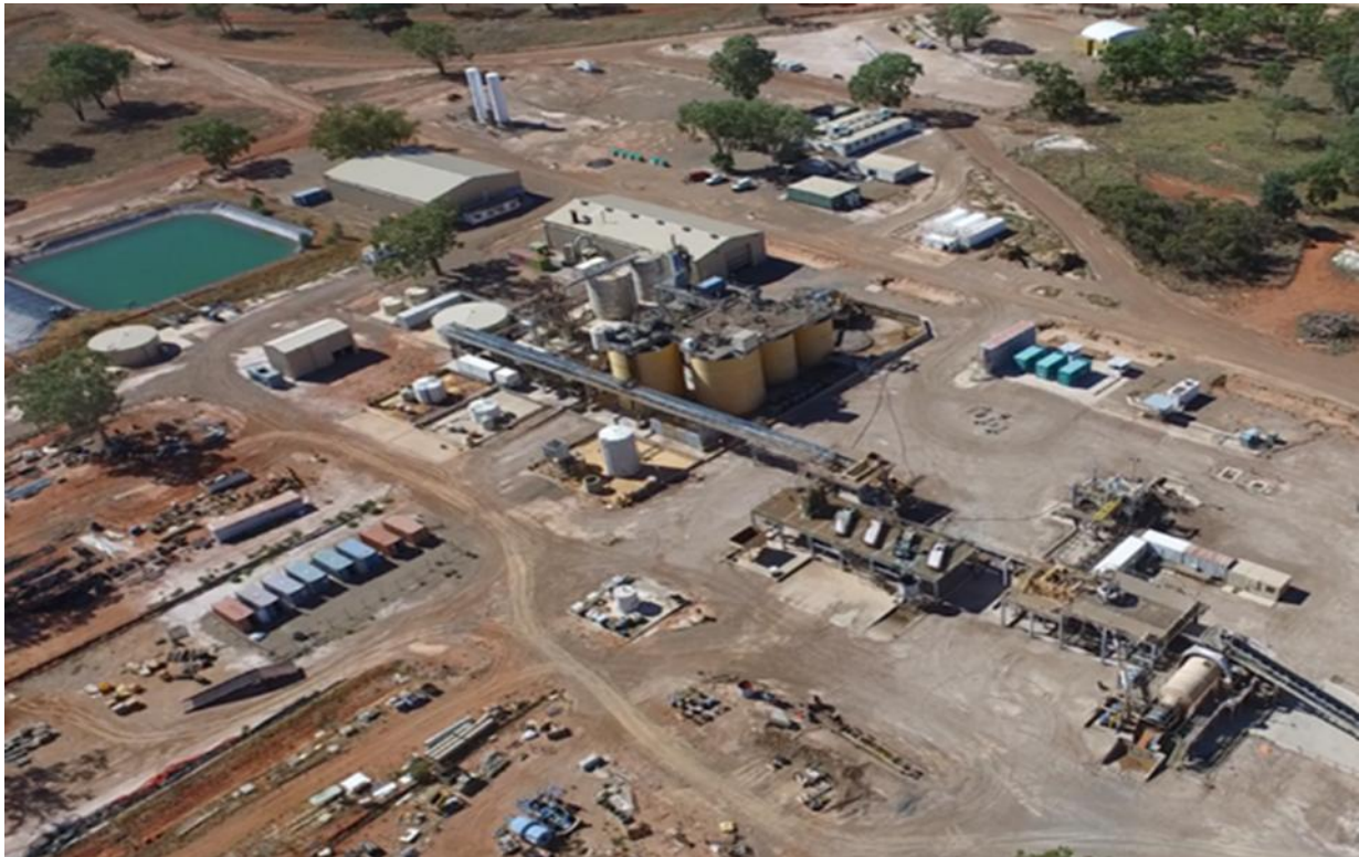
Figure 3: The existing Wonawinta Processing Plant.
