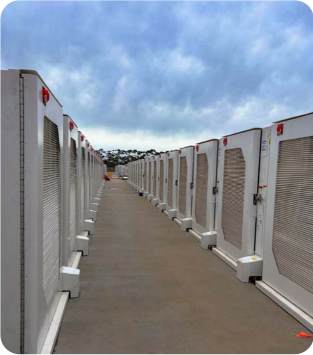
Battery containers at the Mortlake large-scale battery energy storage system.
