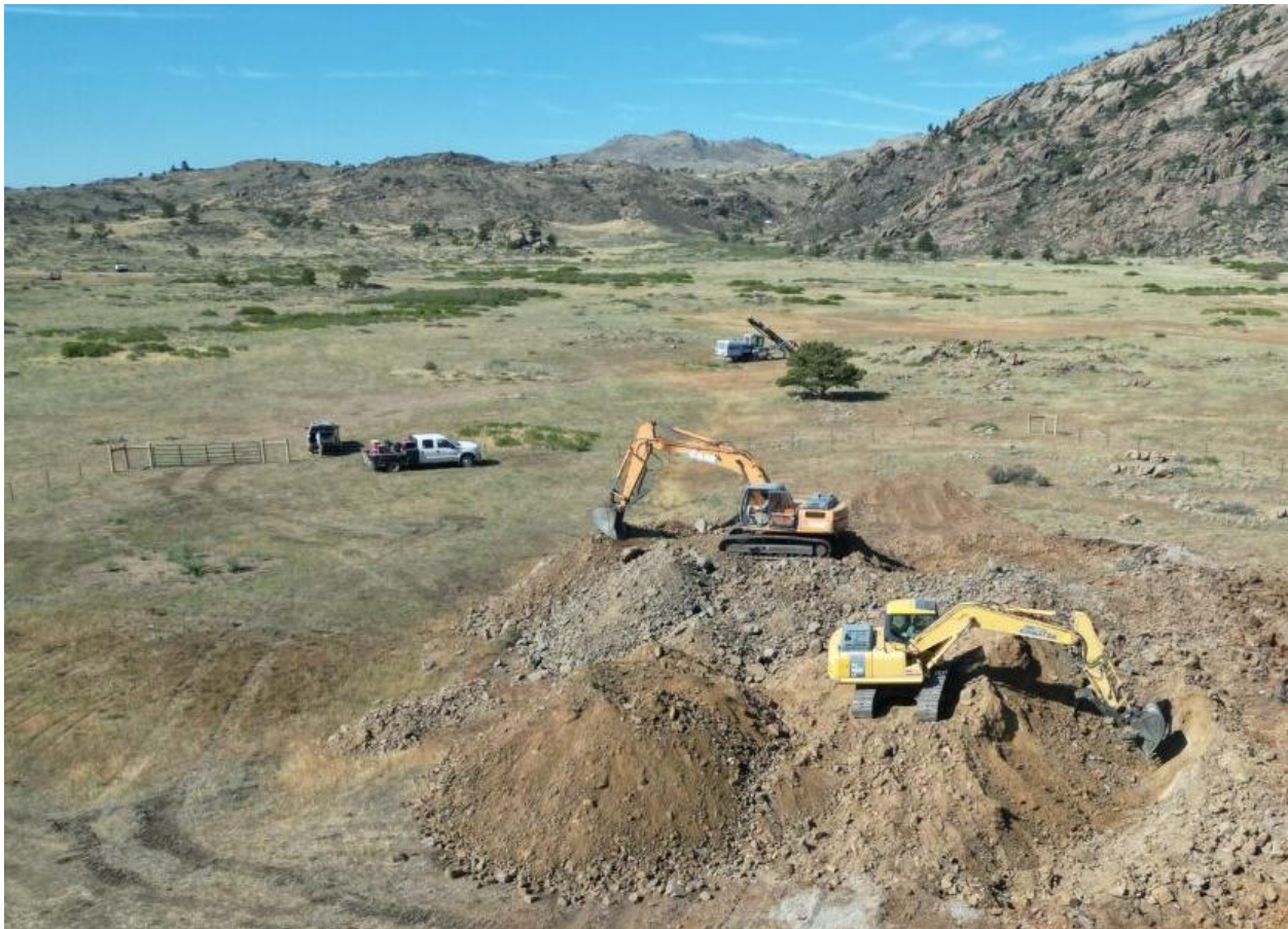
Figure 1 – Aerial view of excavating the blasted, weathered material at the CSM Test Mine
