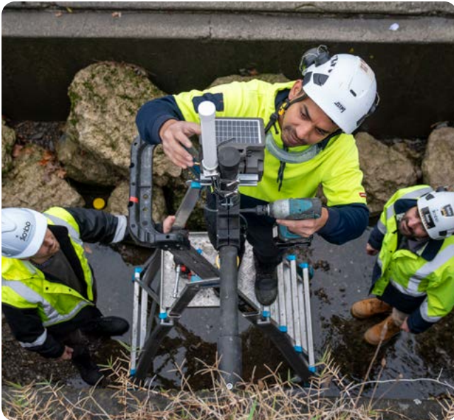
Technicians installing solar-powered sensors in Havelock North.
