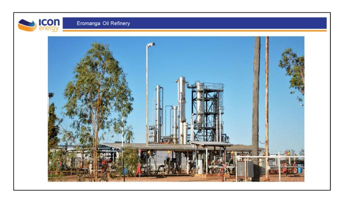
This facility is capable of refining over 2000 BOPD and currently operates on approximately 1100 BOPD.
