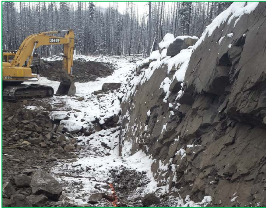
Exposed phosphate rock zone looking south
