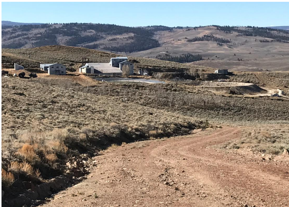
Figure 2. Existing mine infrastructure at Sooner Lucky Strike Mine
