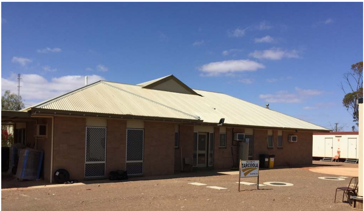
Figure 7: Main accommodation block – refurbished Tarcoola hospital
