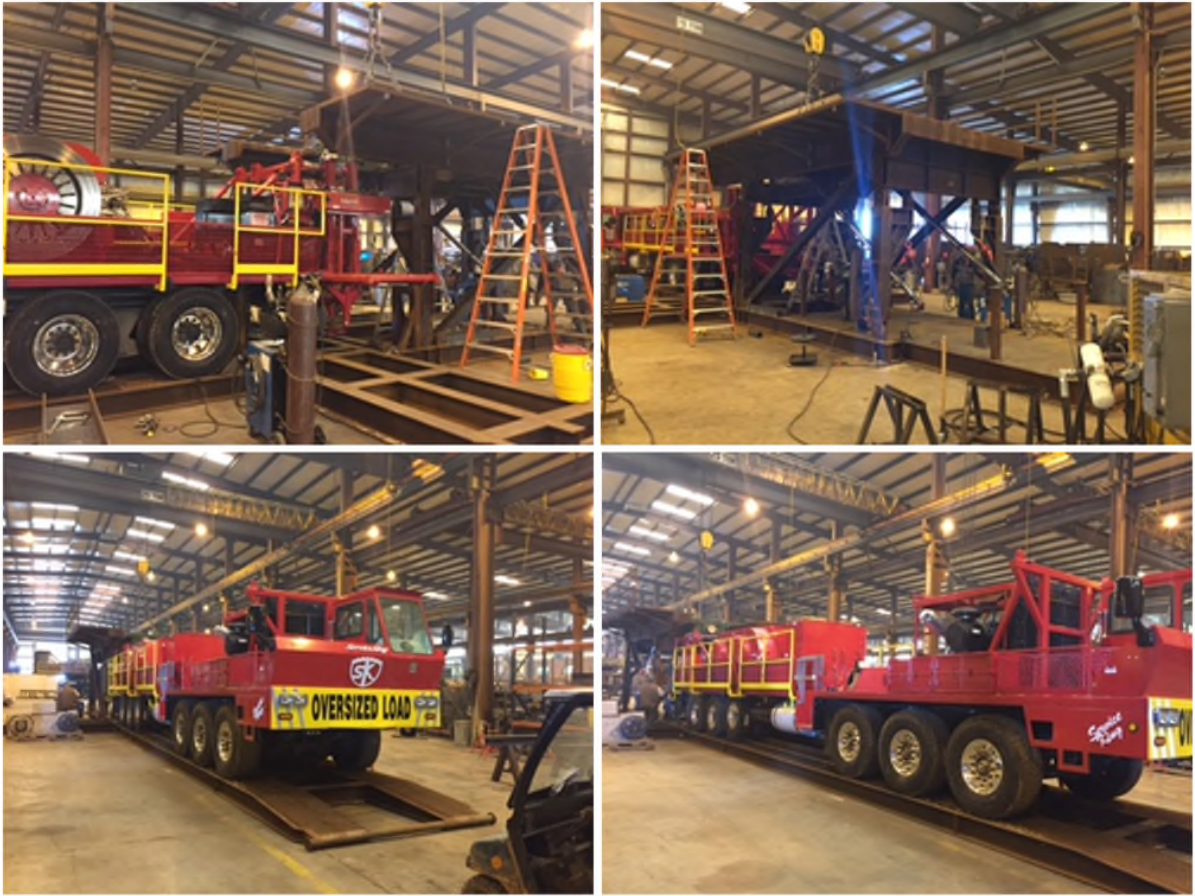
Final fitout and customisation of drilling rig and drilling platform
