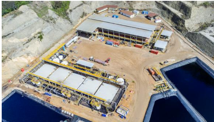
Image 4 – Aerial view of the 25kt SX-EW plant
